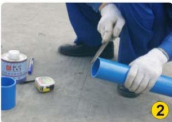
2. Chamfer the cut ends and remove the all burrs from inside and outside diameter of pipe with a knife-edge, file, or deburring tool. Make sure all joining surfaces are free from dirt, dust, water and oil.
