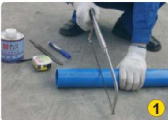
1. If it is necessary, cut the pipe to the desired length with pipe cutters, hacksaw or cross cut saw, make sure the cut is square.
