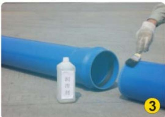
3. Apply lubricant on the spigot end of the pipe and the surface of gasket. The lubricant shall be nontoxic and shall have no deteriorating effects on the gasket and pipe materials.
