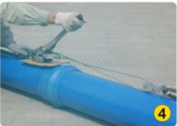
4. Insert the beveled spigot end into the bell with pull tool until it contact with the gasket. Push the spigot end in until the reference mark on the spigot end is flush with the end of the bell. If undue resistance to insertion of the beveled end is encountered or the reference mark does not reach the flush position, disassemble the joint, and check the position of the gasket, and remove any debris.
