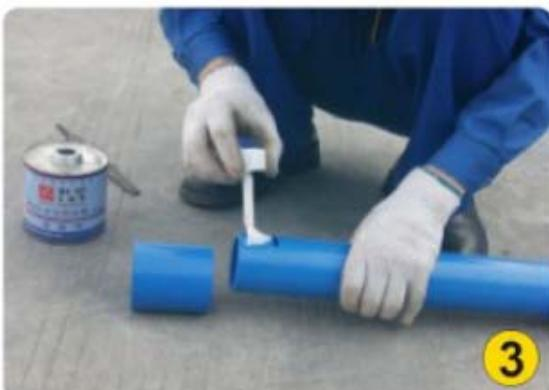
3. Coat the inside of the fittings socket with a medium layer of cement. Immediately apply a full even layer of cement on the pipe for a distance slightly greater than the depth of the fitting socket. If cement dries on either surface before joining, apply another coat.
