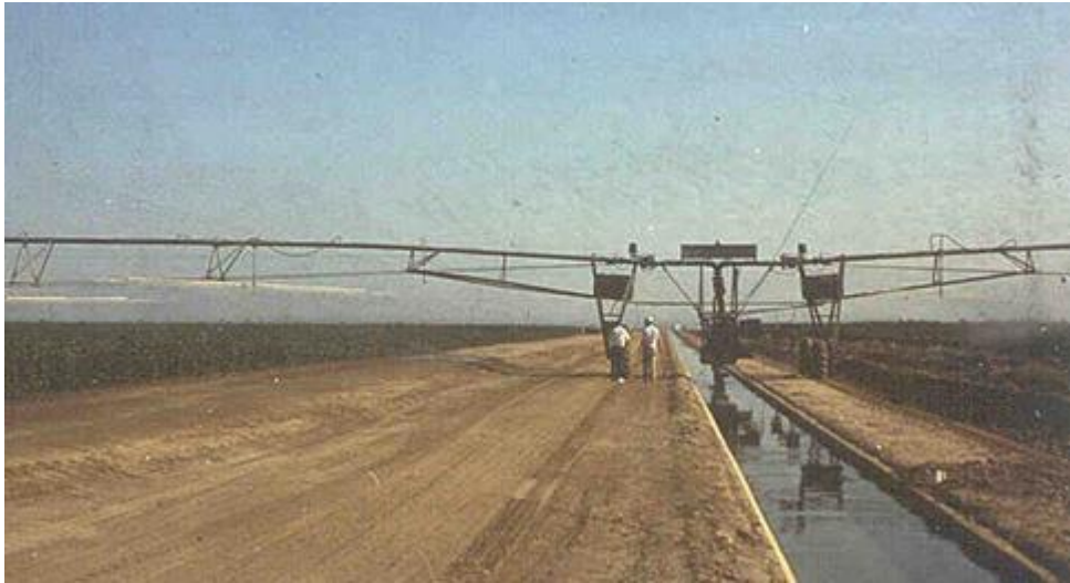
Figure 5. A Linear Move system. Notice the concrete water supply channel (and the fact that the system spans both sides of the channel).
